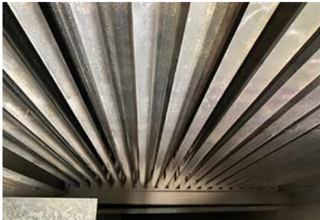
Figure 5: Condenser inspection during fall 2020.
