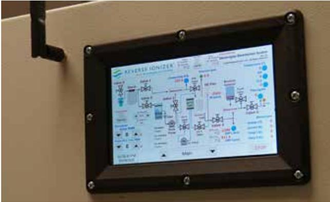
**Figure 2: Plasma/copper-silver ionization unit and oxidizing biocide generator.**
